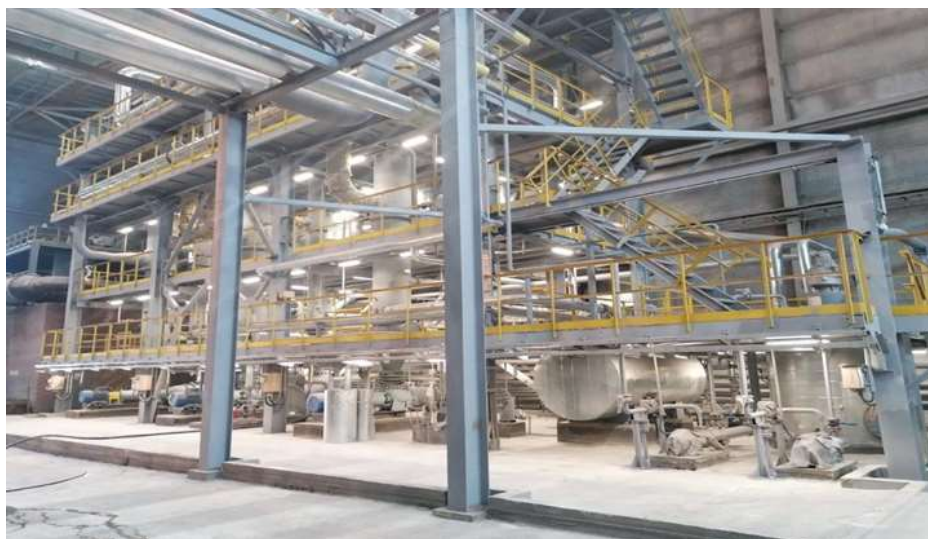
Figure 6. Soda-sulphate mixture production facility at Krasnoyarsk aluminium smelter.
